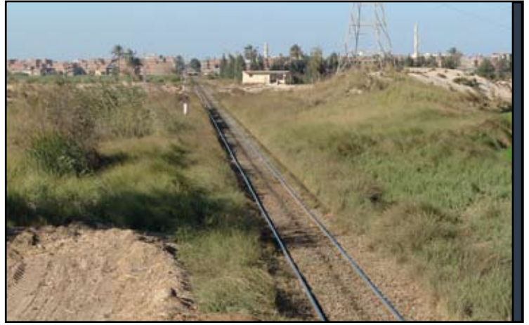
Al-Marg - Shibin al-Qanatir railway dividing the site into two parts
